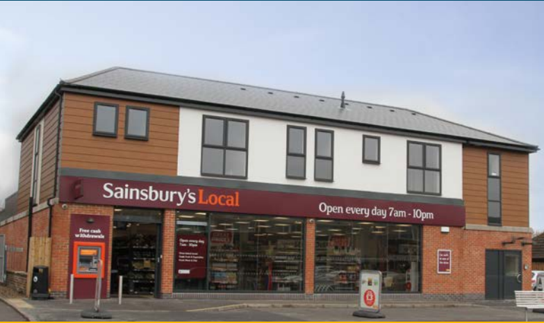
CONVENIENCE FOOD STORE AND APARTMENTS, WOLLATON, NOTTINGHAM
